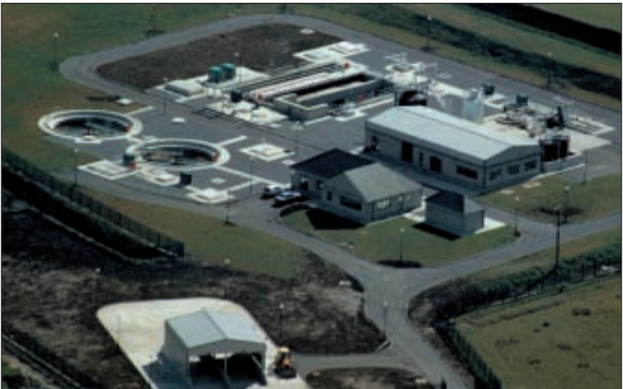
Loughrea Sewerage Scheme
