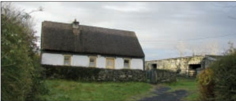
Thatched house in Kinvara which is a Protected Structure
