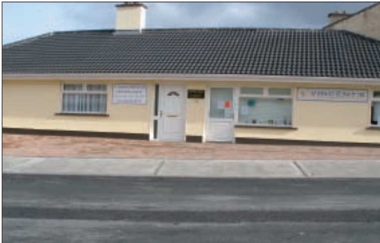
The St Vincent de Paul building extension in 2007 on Jubilee Street in Ballinasloe was core funded through the Ballinasloe RAPID Programme
