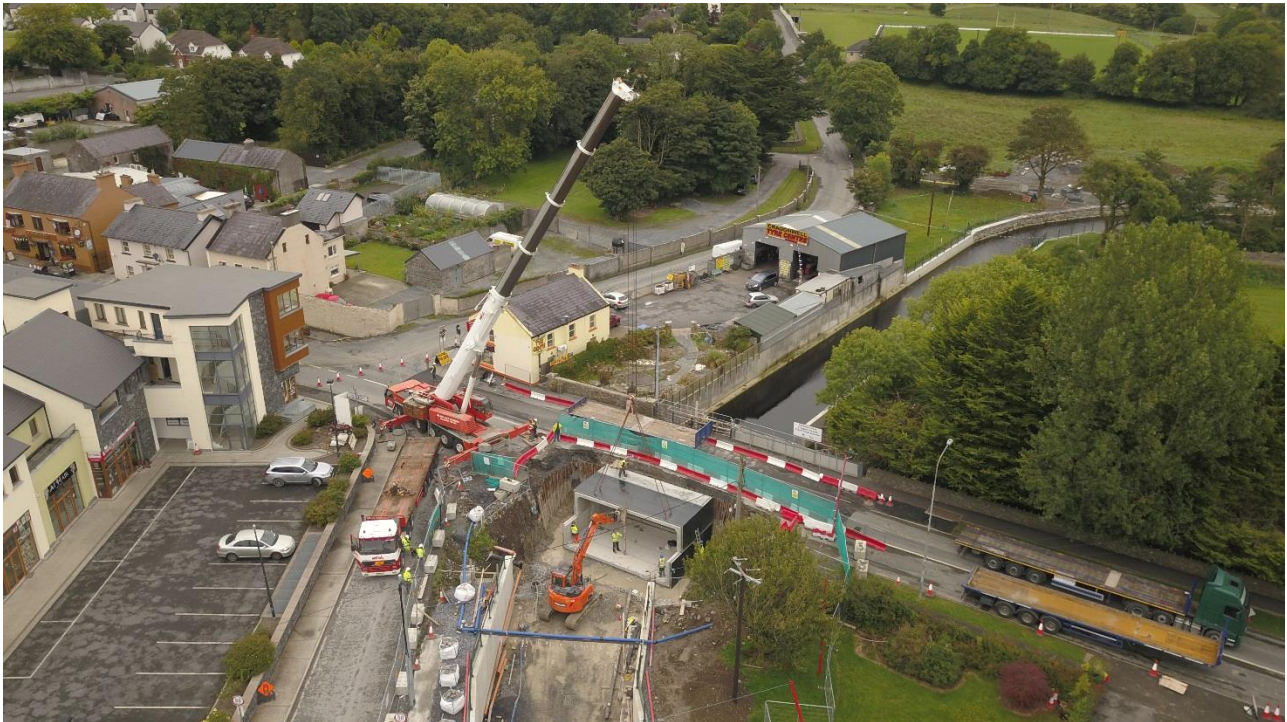
Figure 1; Aerial View of Bridge Replacement
