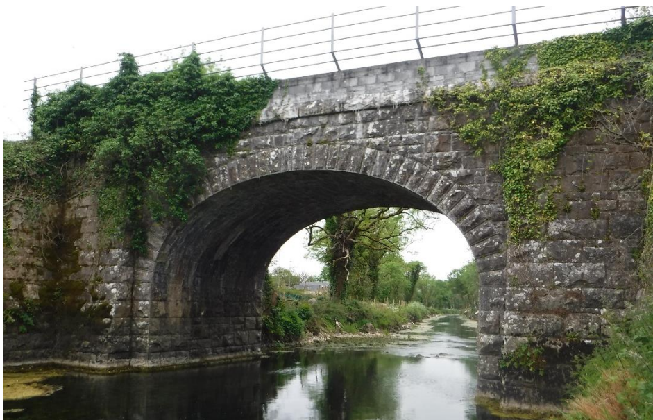
Figure 4; UB154 Railway Bridge
