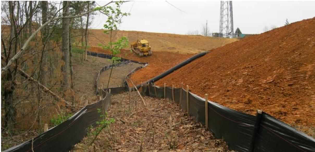
**Figure 5.2: Typical Temporary Settlement Pond**
