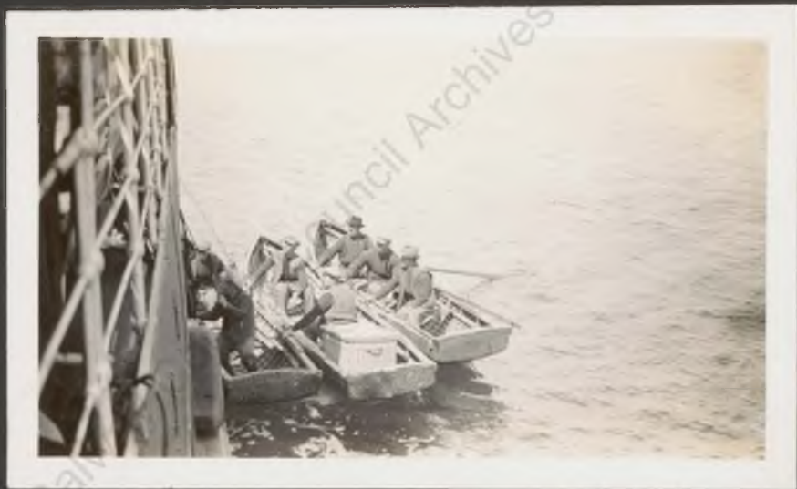
LANDING STORES INISHMAAN
