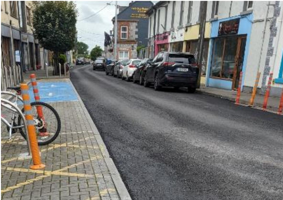
FIG.7 – CROSS STREET CARRIAGEWAY SEALING
