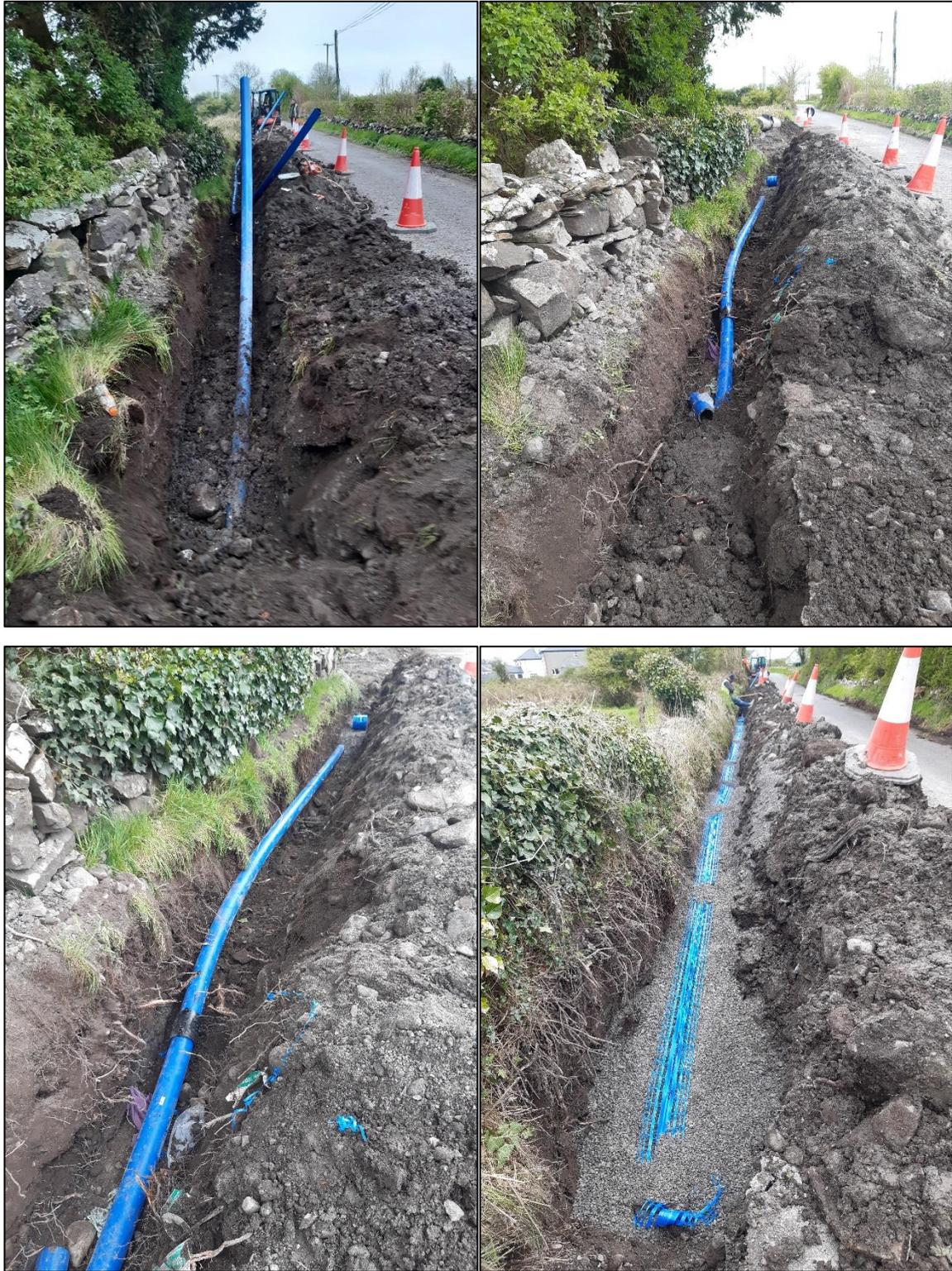
**FIGURE 3 & 4.** OPEN CUT EXCAVATIONS AND TRENCH REINSTATEMENTS ON THE BULLAUN ROAD.
