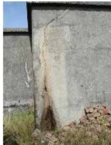
Photograph 3-6: Leaking Reservoir.
