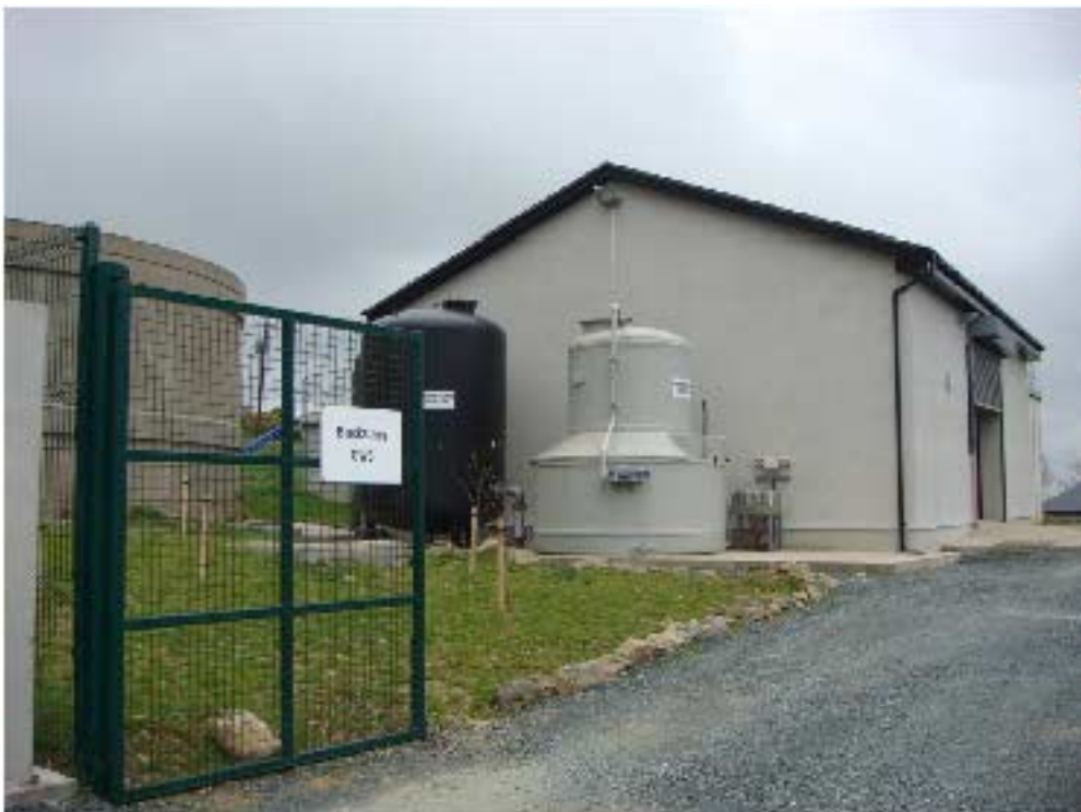
Photograph 2-2: Blackstairs Group Water Scheme (Co. Wexford) which was part of the Leinster DBO bundle completed in 2010.
